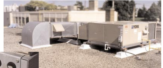
Curb-mounted isolation springs keep the HVAC units raised above the rooftop, minimizing the transference of noise and vibration to the church interior.
